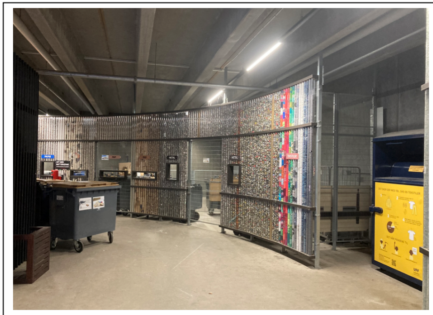
Image 1. Example of a waste management / recycling / storage area in an apartment scheme.
